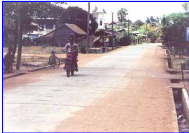
Image 3 – Bamboo Reinforced Concrete Paving
