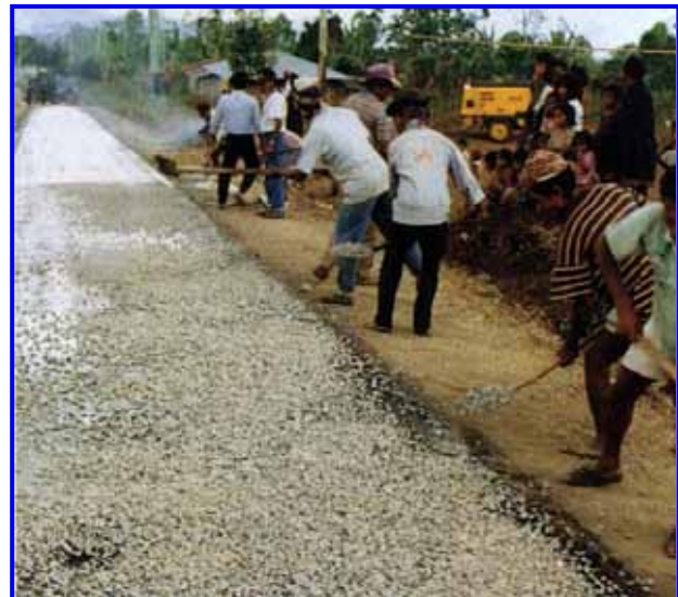
Image 4 – Hand Laid Bituminous Surface Dressing
