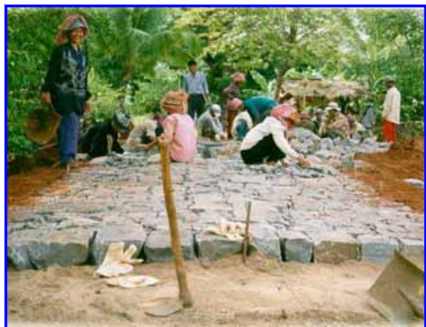
Image 2 – Dressed Stone Paving under Construction
