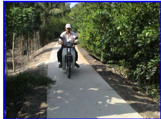
Figure 1, above left, shows an inappropriate over-provision of road width for a LVRR. This road will incur high maintenance costs. Figure 2, above right, shows a 1.4 metre wide concrete, all-weather, low maintenance VLVR suitable for the predominant 2 wheeled vehicles using the route, allowing safe passing of loaded vehicles.
