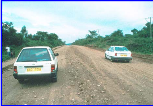
Figure 1, above left, shows an inappropriate over-provision of road width for a LVRR. This road will incur high maintenance costs. Figure 2, above right, shows a 1.4 metre wide concrete, all-weather, low maintenance VLVR suitable for the predominant 2 wheeled vehicles using the route, allowing safe passing of loaded vehicles.
