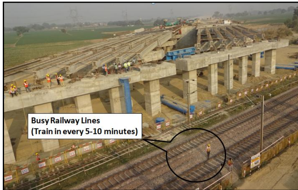
FIGURE 2 Actual site photograph
