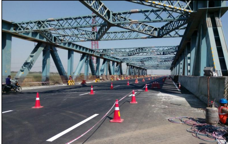
FIGURE 20 Photograph of completed truss
