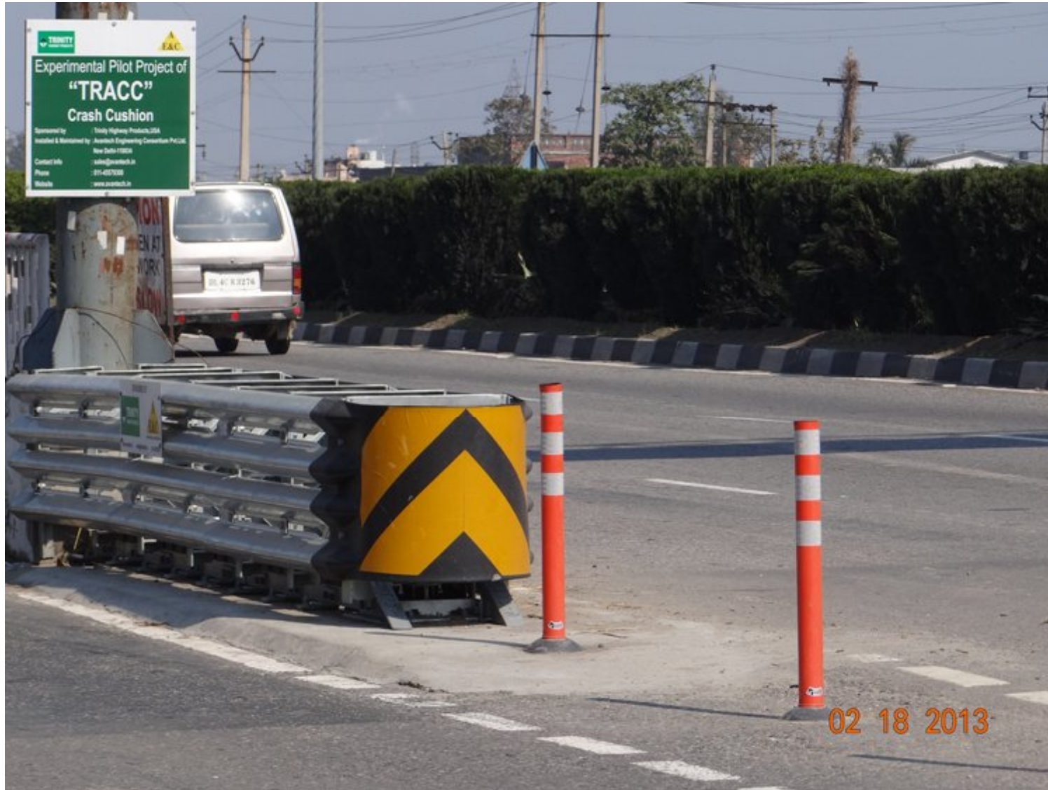
Crash Cushion at L&T-IDPL's, 6 Lane, 10 KM long Elevated Corridor on NH-1
