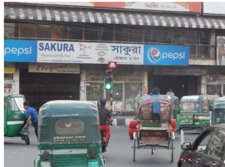
Installed traffic signal with countdown timer
