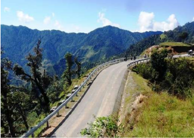
W-beam crash barrier installation along cliff side Khodpe Bajhang Road
