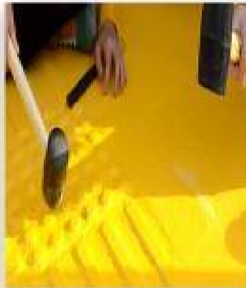
Applying on Pavement
