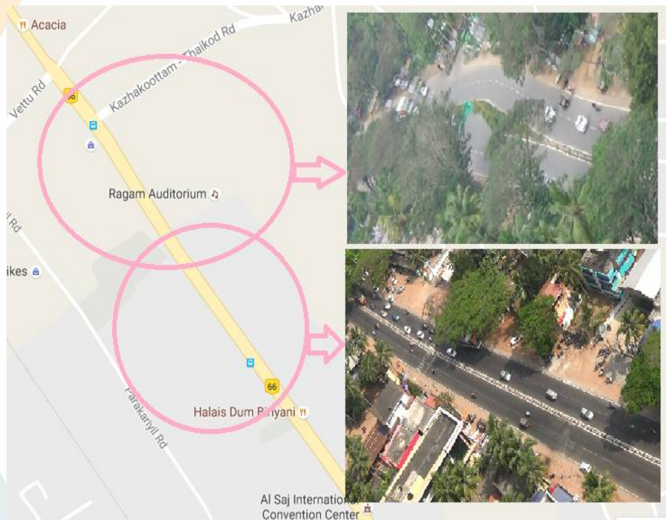
Study stretch at Vettu Road Junction, Trivandrum, Kerala
