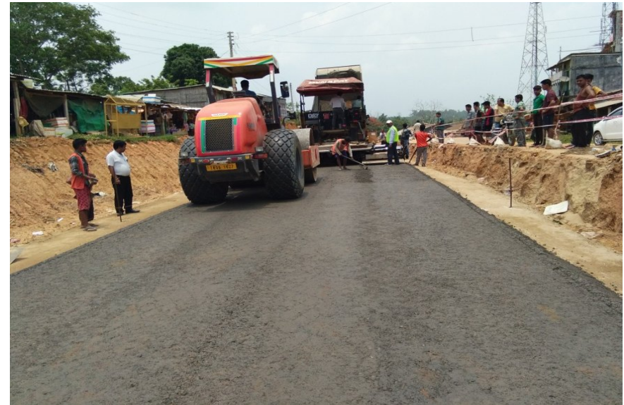
Laying and Compaction of Foamed Stabilized Mix
