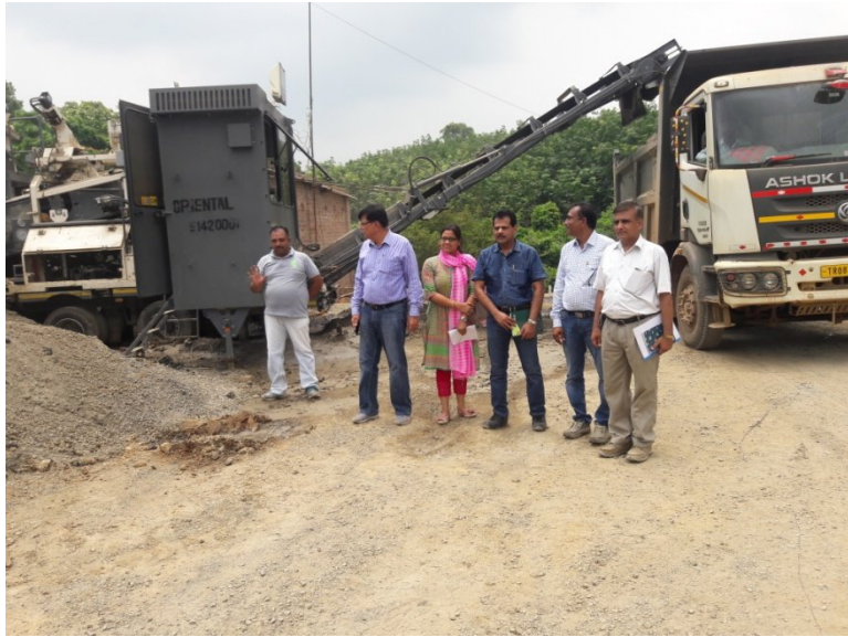
Collection of Foamed Stabilized Mix from Plant
