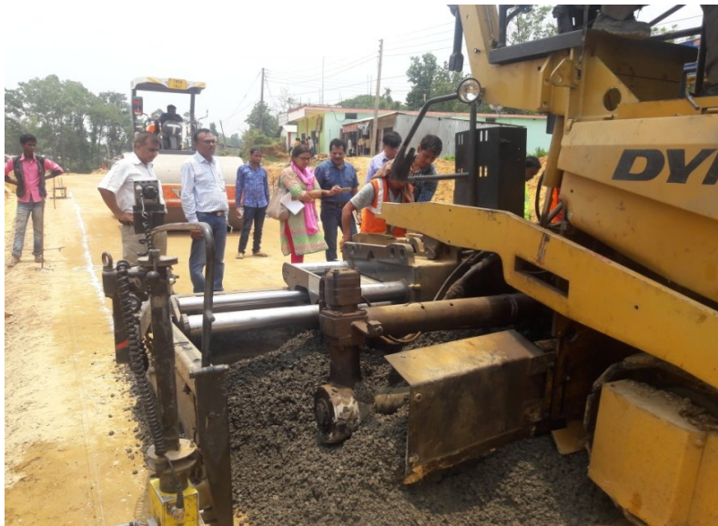
Close view of Foamed Stabilized Mix
