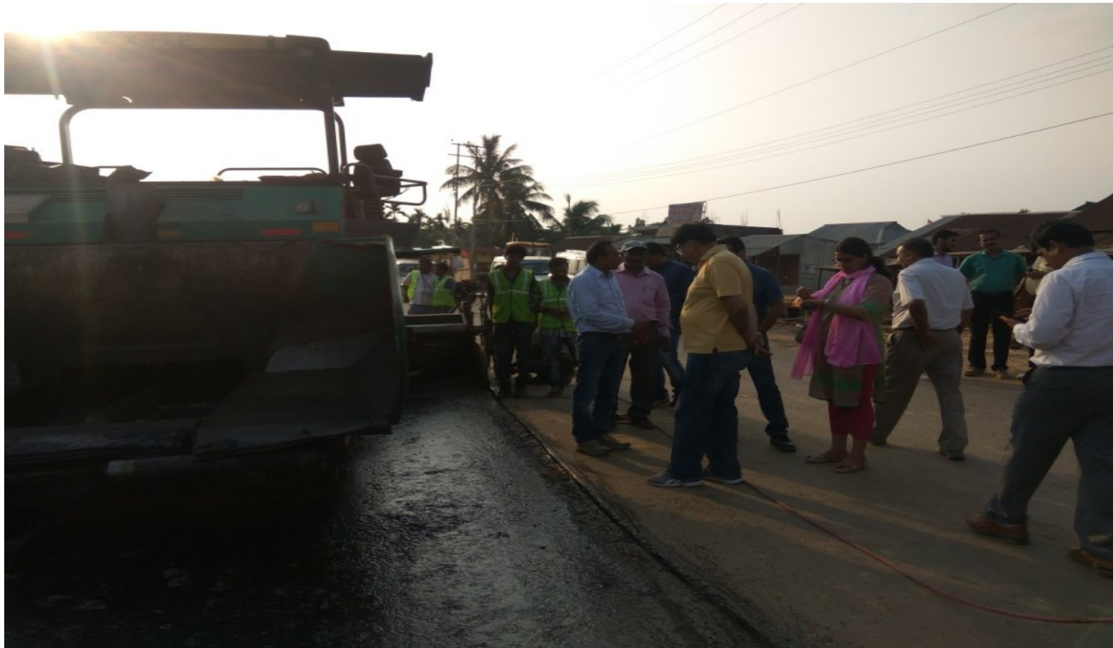
Application of Tack Coat on BSM Layer before laying of BC
