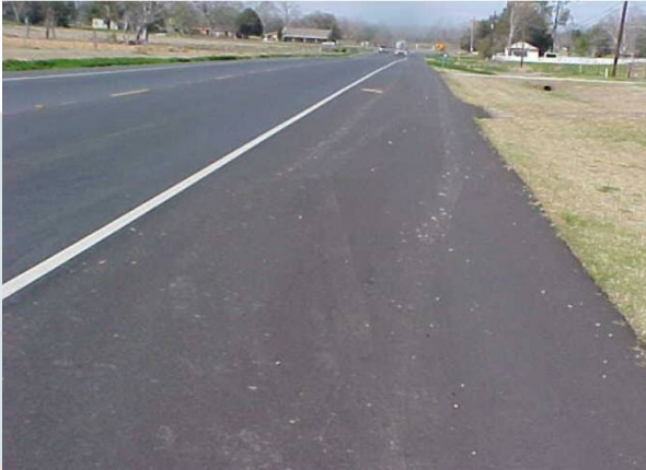
Condition 5. No contiguous drop-off, which is in excess of 2 inches, along the roadway. Vehicles and travelers experience no discomfort while pulling onto and off the shoulder.
