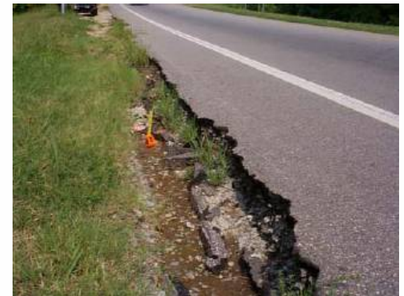
Condition 1. Contiguous drop-off in excess of 2 inches stretching for more than 1/2-mile along the roadway. Driver might lose control of the vehicle
