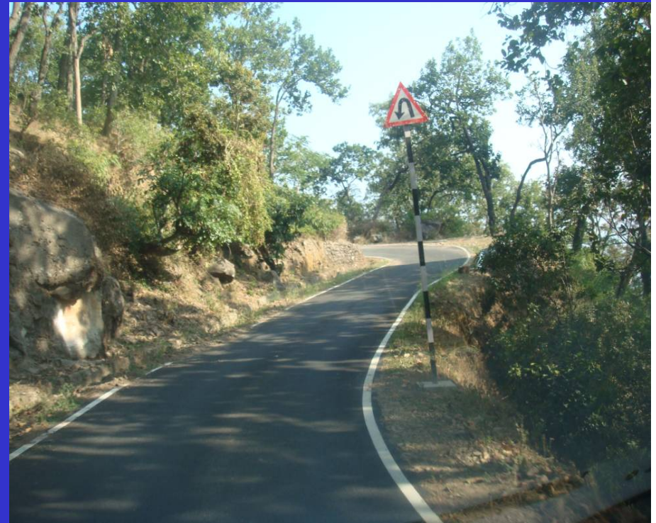
Warning signs are posted very close to the sharp blind curve at higher level
