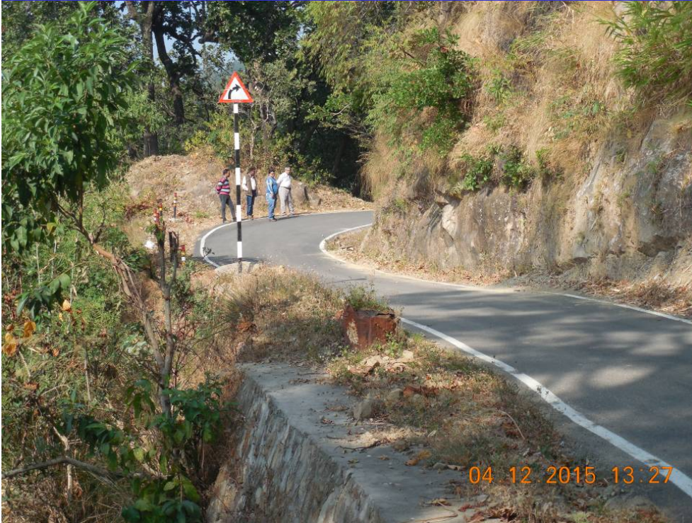
Warning signs are posted very close to the sharp blind curve at higher level
