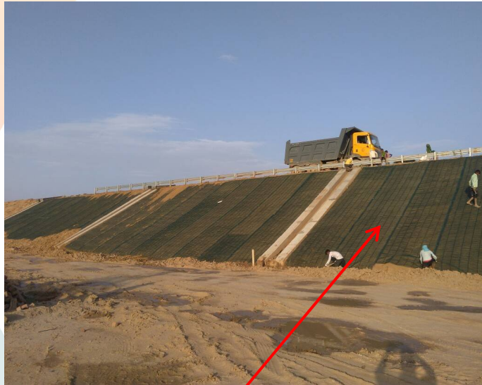
Multimat in slope protection with turfing
