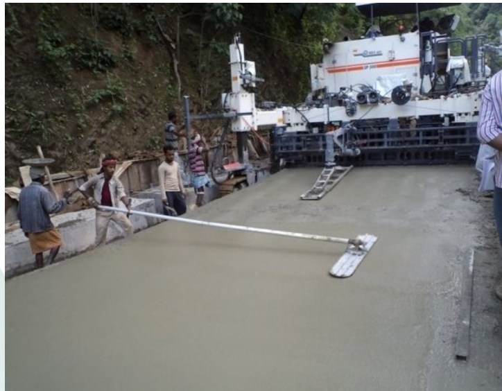
CCP laid with 5 m Custom-made paver
