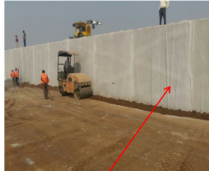
Geo Composite for internal drainage of soil
