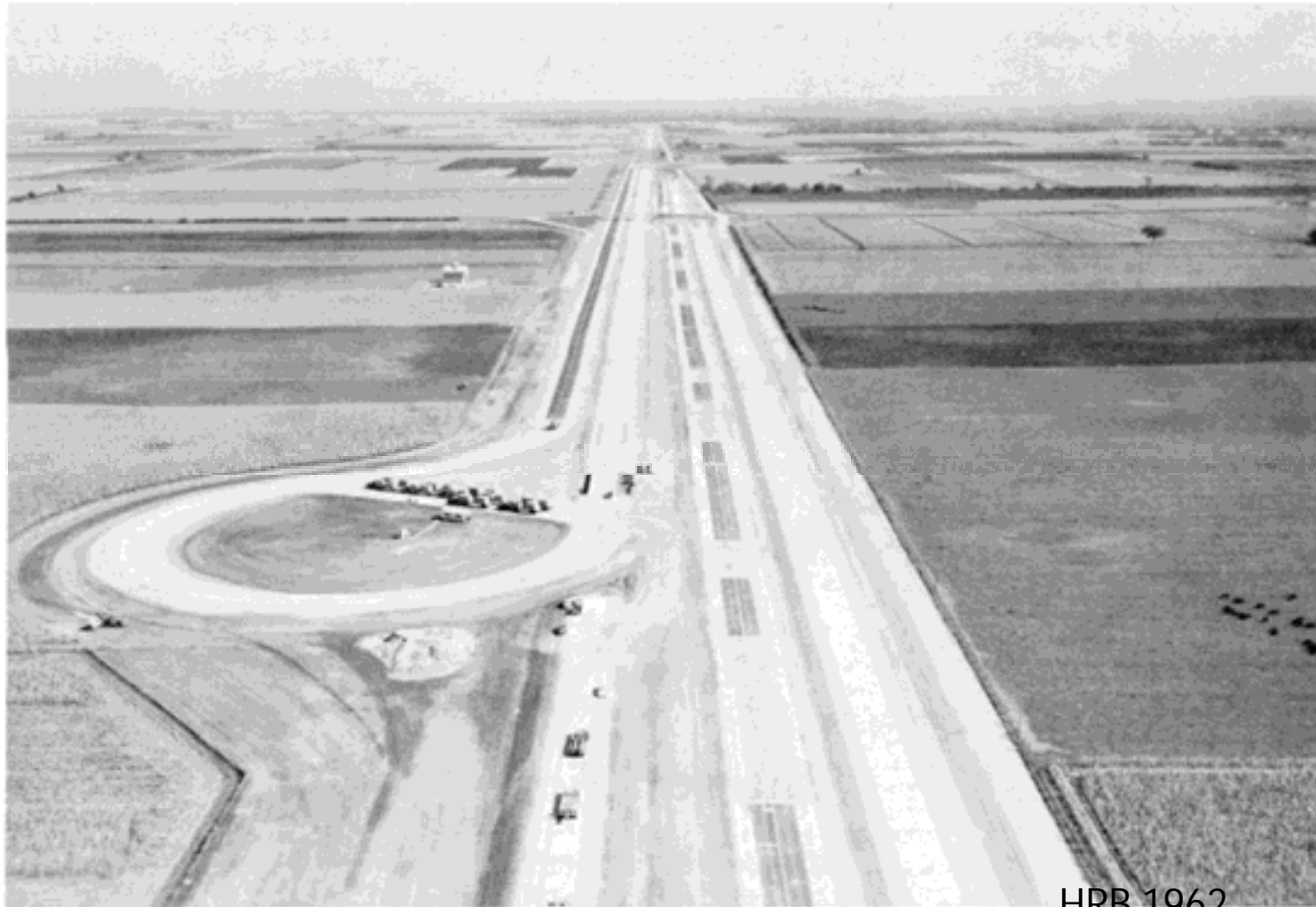
Figure 1. Looking east, Loops 5 and 2 in foreground.
