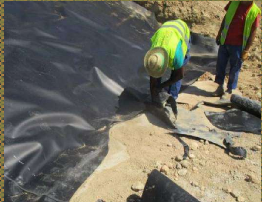
Remodeling and clean-up of the sheet on the foot of the slope
