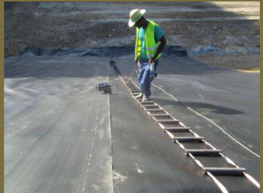
Execution the welded joints in the slope
