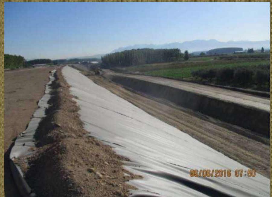
General view of the execution of the shoulders
