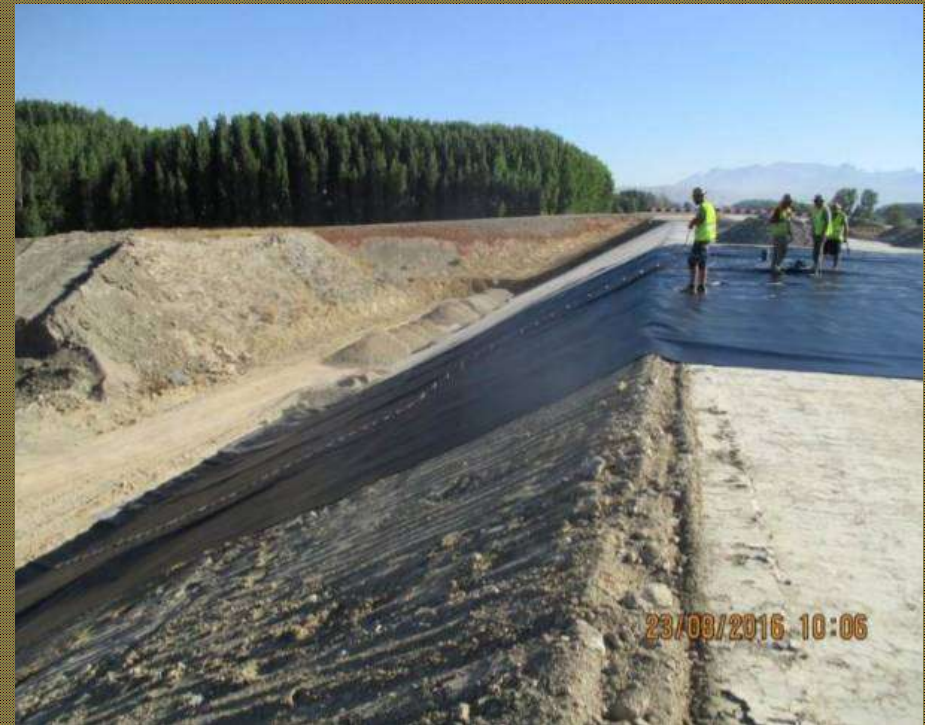
Placement of the sheet on the slope
