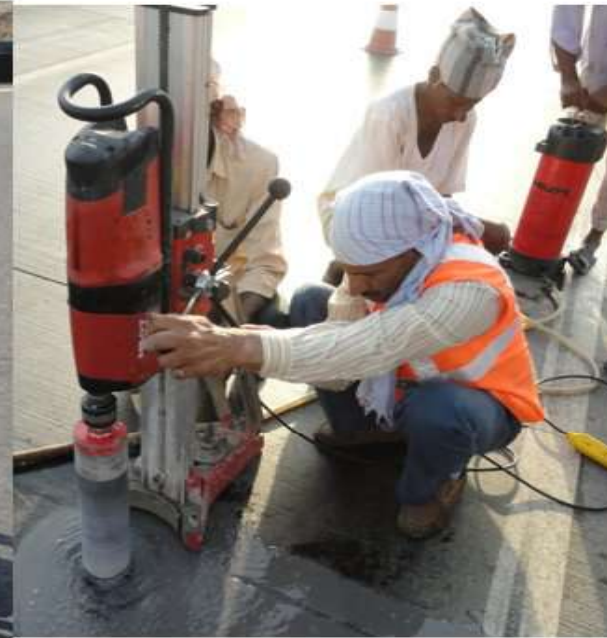
(B) Core Extraction on CC Pavement
