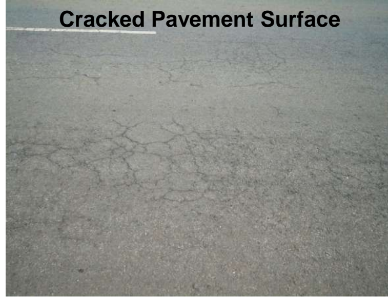
Cracked Pavement Surface
