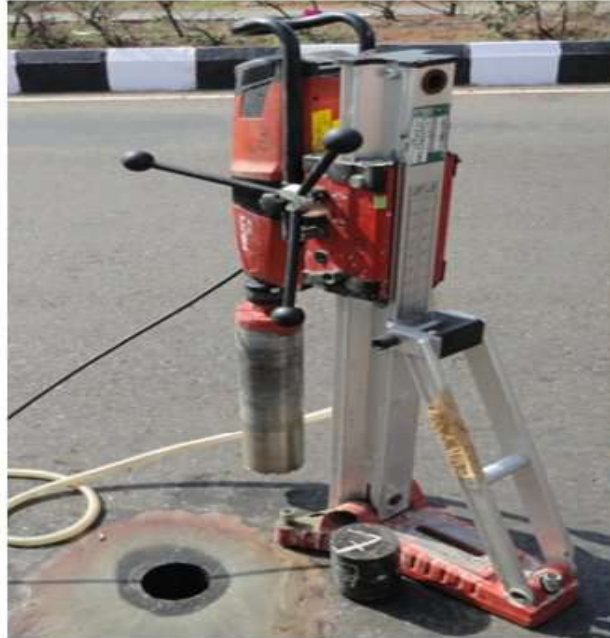
(A) Core Extraction on Bituminous Pavement
