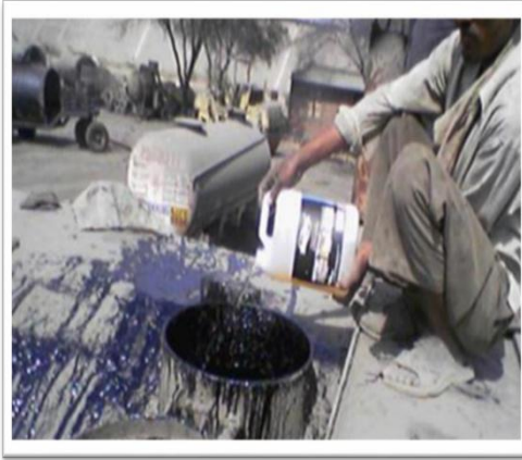
Organosilane mixing in bitumen
