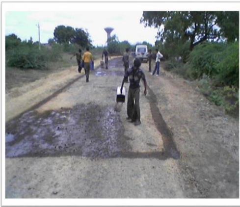
Prime coat with Organosilane
