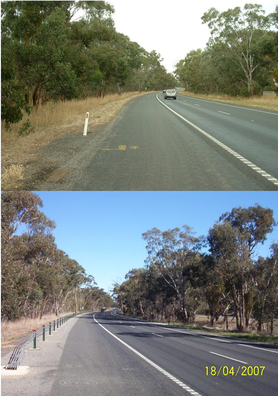
FIGURE 3 Before and After Treatment Wire Rope Safety Barriers
