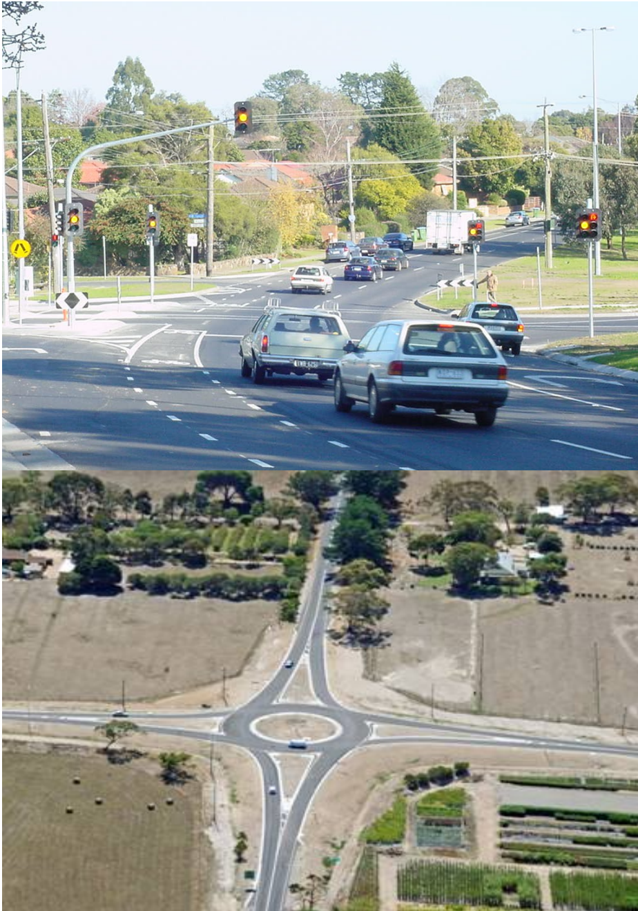
FIGURE 2 Before and After Intersection Treatments: New Traffic Signals And Roundabout
