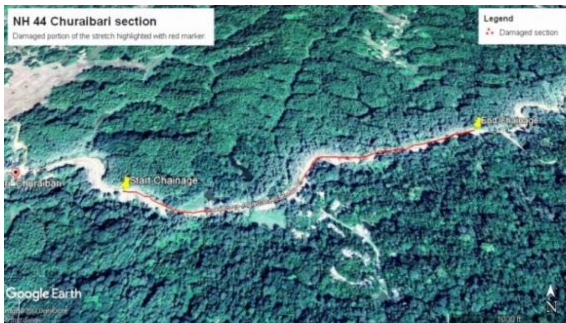
FIGURE 2(a) Damaged stretch through the dense forest
