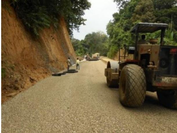
FIGURE 6(c) Granular base being compacted
