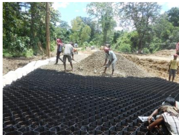
FIGURE 6(b) StrataWeb® geocells being infilled with graded aggregate
