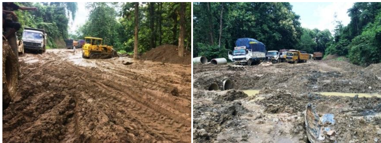
FIGURE 2(b) Actual site condition
