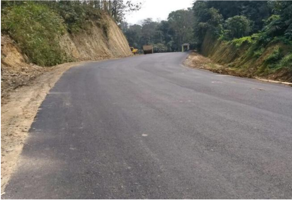
FIGURE 8 Finished asphalted surface
