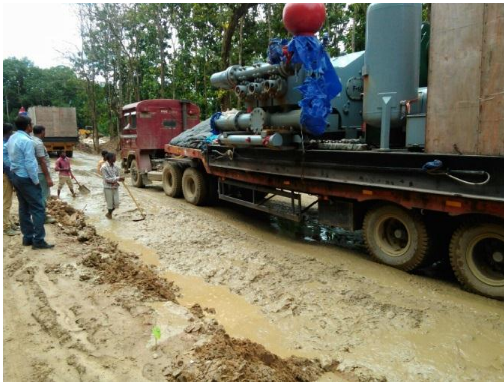
FIGURE 7 Continuous traffic movements over geocells during monsoons
