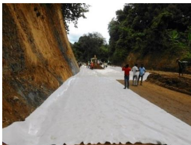
FIGURE 6(a) Laying of Nonwoven geotextile on dressed subgrade
