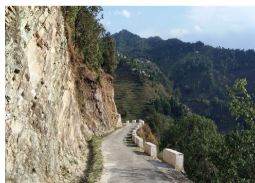
Status of off-carriageway road after maintenance by MMD members
