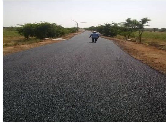
Image-8, completed CGPC road
