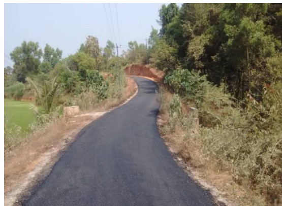
Image-12, completed CGPC road
