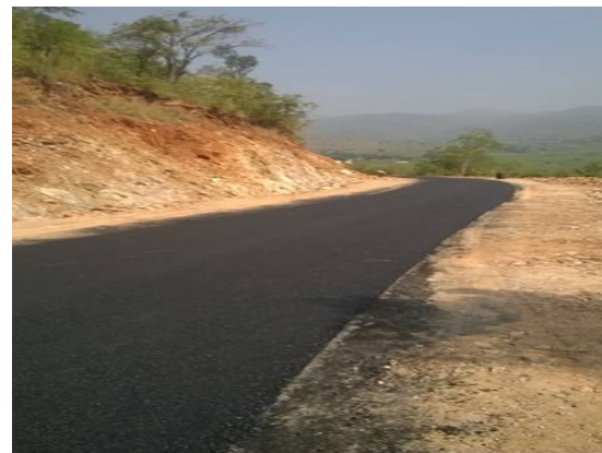
Image-10, completed CGPC road
