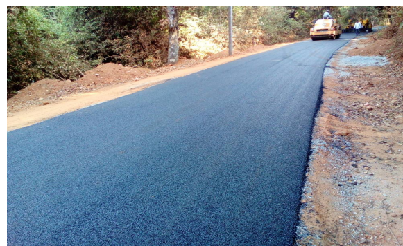
Image-14, completed CGPC road
