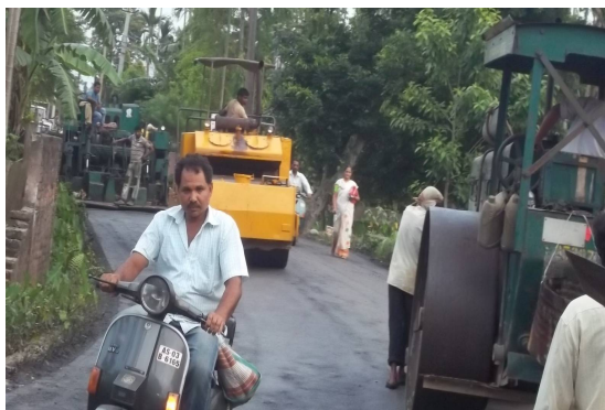
IMAGE 14 laying & compaction cold mix SDBC
