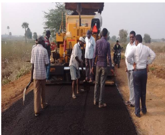
IMAGE 12 laying of cold mix MSS
