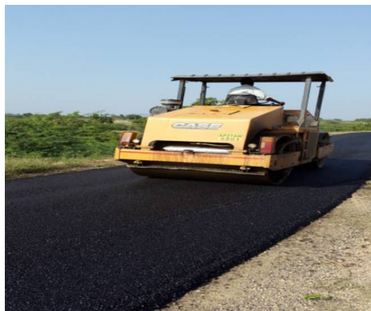
IMAGE 13 compaction of cold mix MSS
