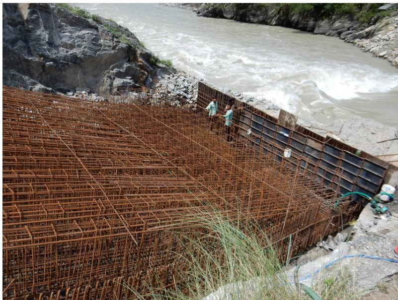
FIGURE 7 Placement of foundation reinforcement cage in progress
