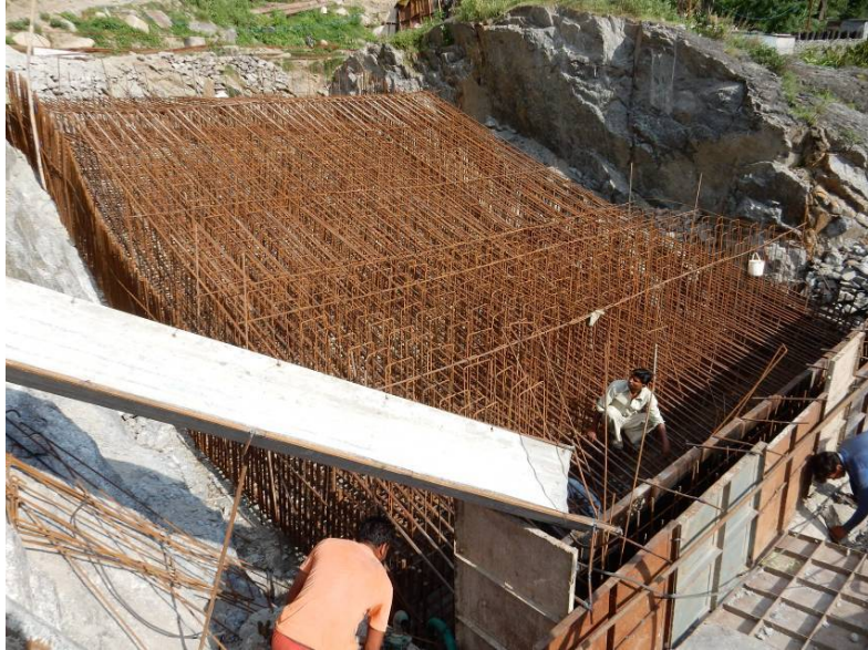
FIGURE 8 Placement of foundation reinforcement cage in progress
