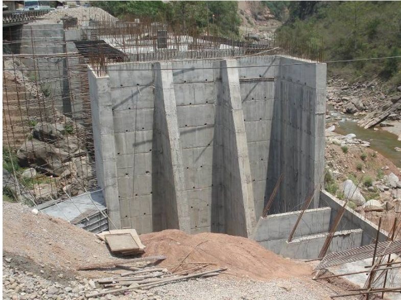
FIGURE 5 Counterfort type abutment
