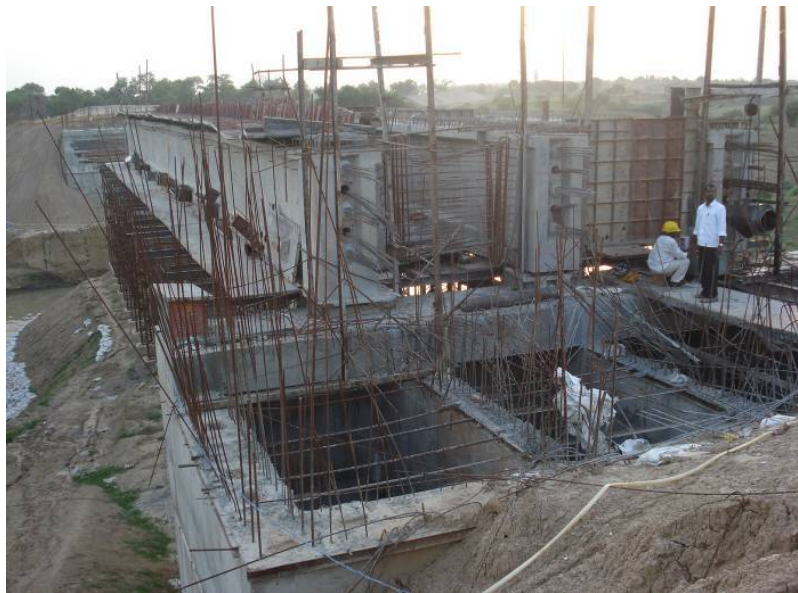
FIGURE 6 Box type abutment
