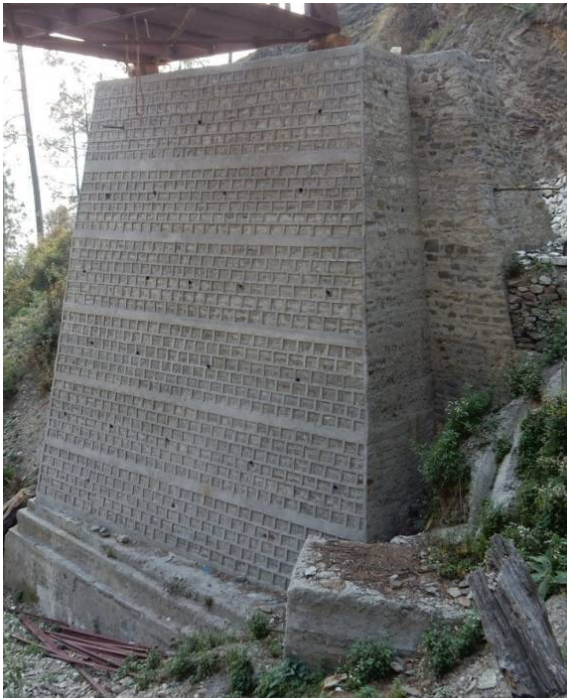
FIGURE 3 Stone masonry abutment
