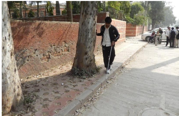
FIGURE 1 Inadequate footpath width
