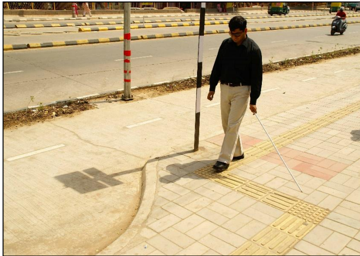
FIGURE 13 Continuous tactile pavers on entire 5.8km BRT corridor
