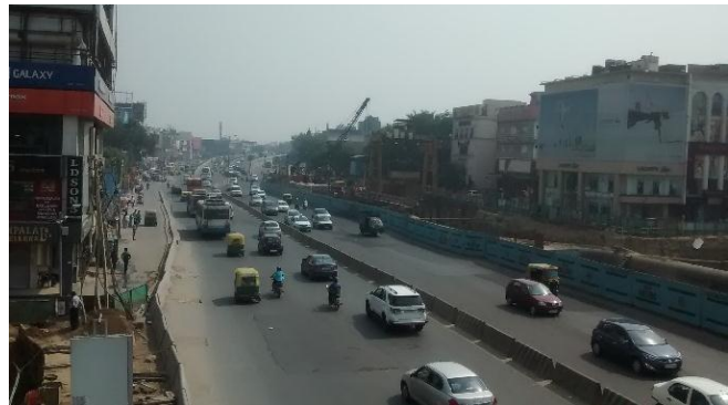
FIGURE 2 Encroachment due to construction on both sides of a road
