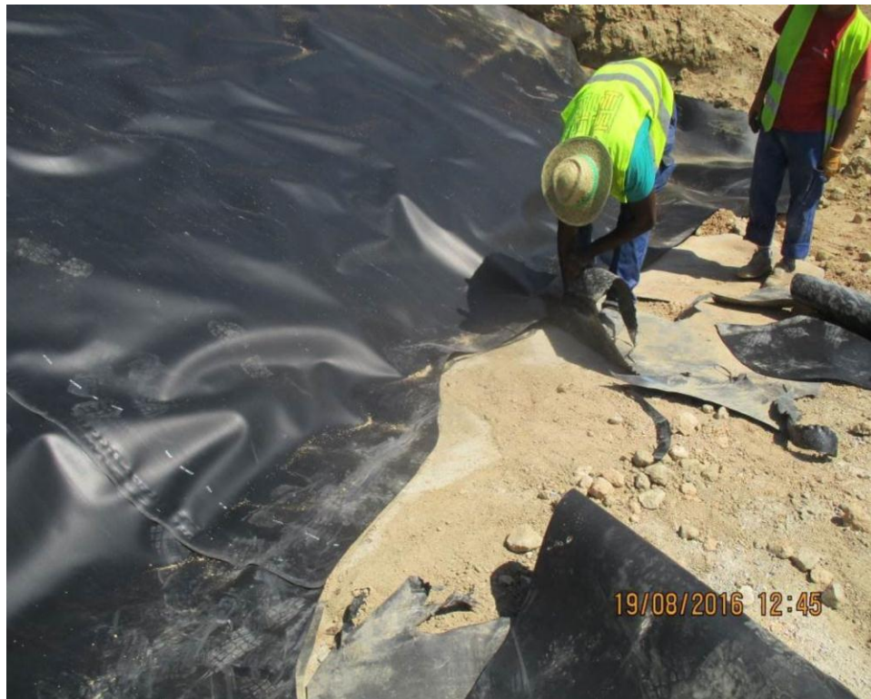
Figure 8 Remodeling and clean-up of the sheet on the foot of the slope
