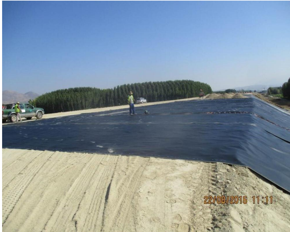
Figure 6 Execution the welded joints in horizontal
