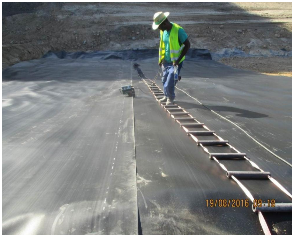
Figure 7 Execution the welded joints in the slope
