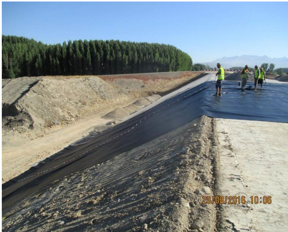
Figure 5 Placement of the sheet on the slope
