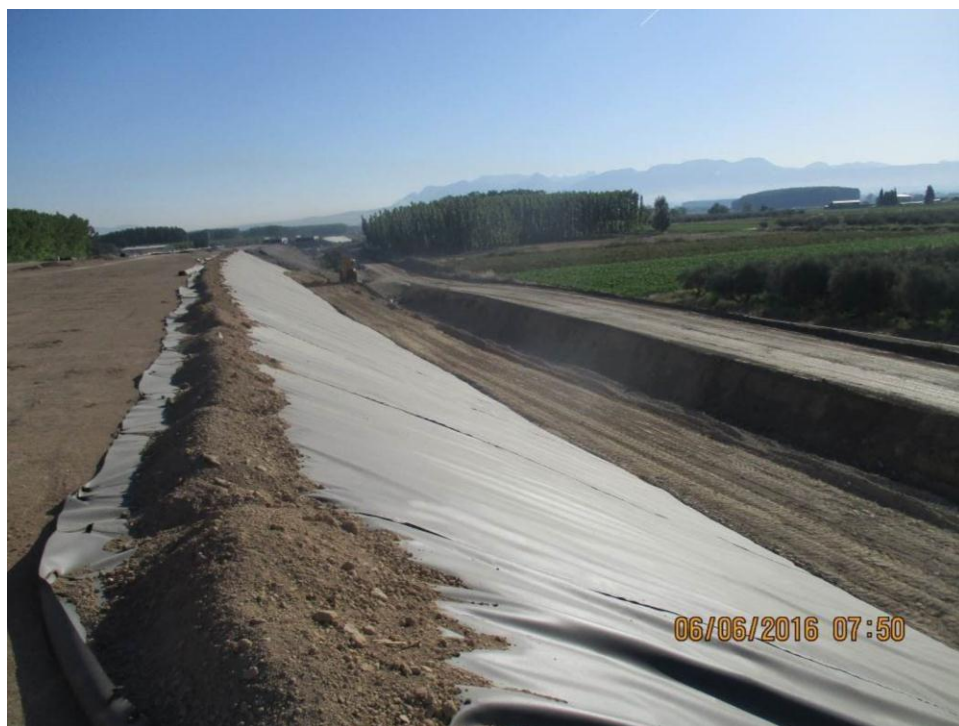
Figure 9 General view of the execution of the shoulders
