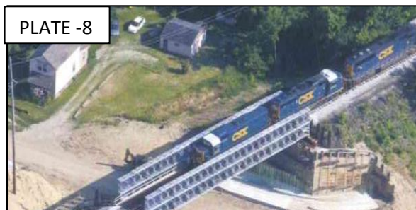
A Rail Bridge with the same equipment.
