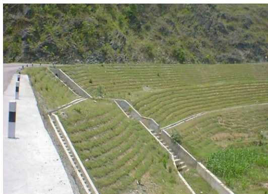
FIGURE 2 Spoil and drainage management
