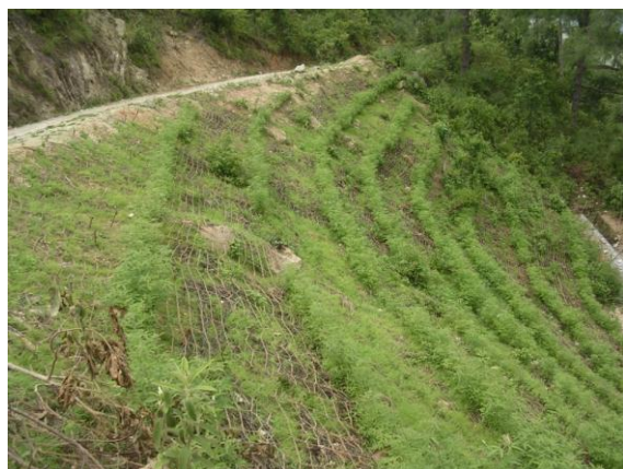
FIGURE 3 Jute netting and brush layering
