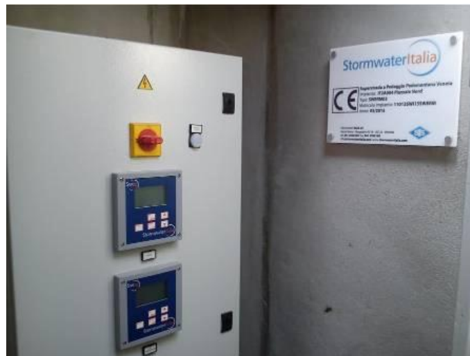
FIGURE 12 Example of local control panel with transmission module
