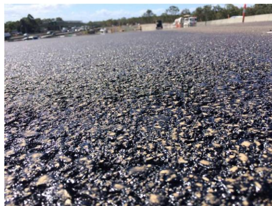
EME first major project in Australia in Brisbane
