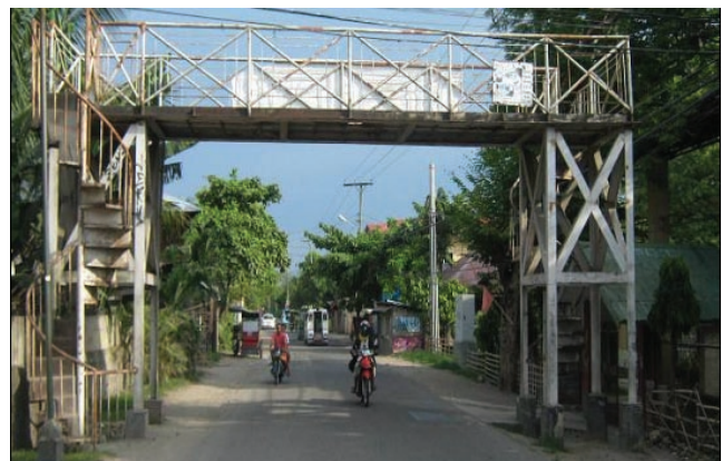
Pedestrian overpass in a relatively low vehicle traffic area on a two lane road in Cebu city. Infrastructure for whom?
