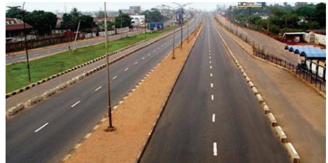
Plate 1: Segregated route way (Courtesy: LAMATA)
