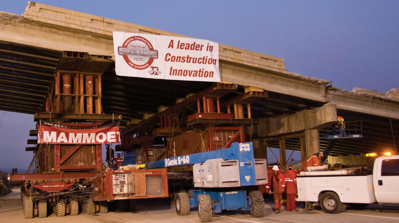
Lifting the old bridge out.
