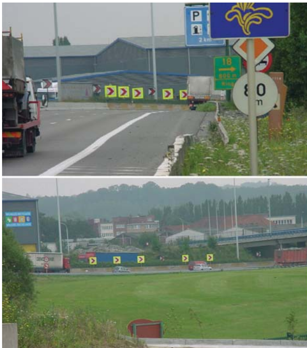
Belgium - Brussels Ring Upgrading
