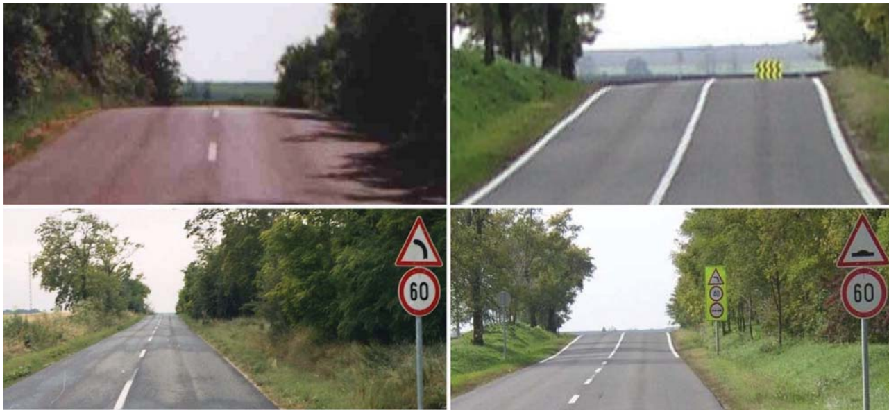
Effect of re-signing - only one accident has occurred since the implementation of the changes.
