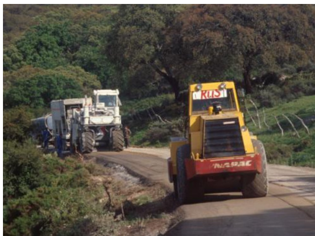
Compaction of recycled material
