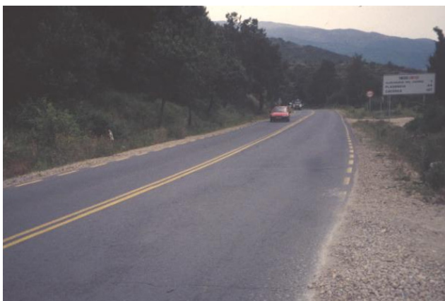
N-630 (Spain) - Recycled pavement in service
