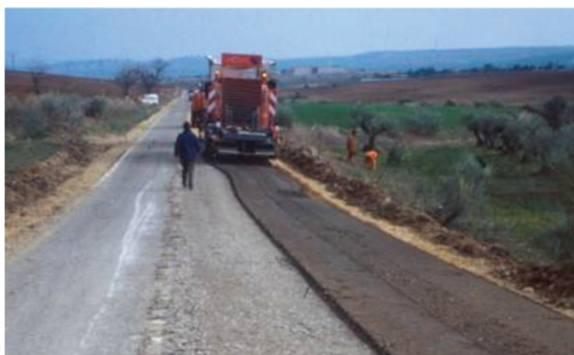
Recycling of a degraded pavement
