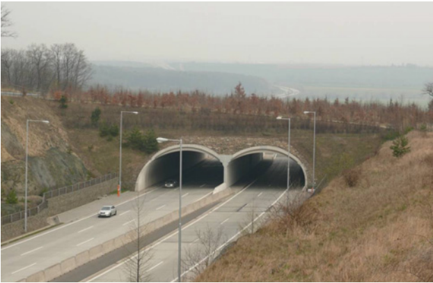
Ecoduct on motorway R35, first construction for wildlife crossing in the Czech Republic, built in 1999
