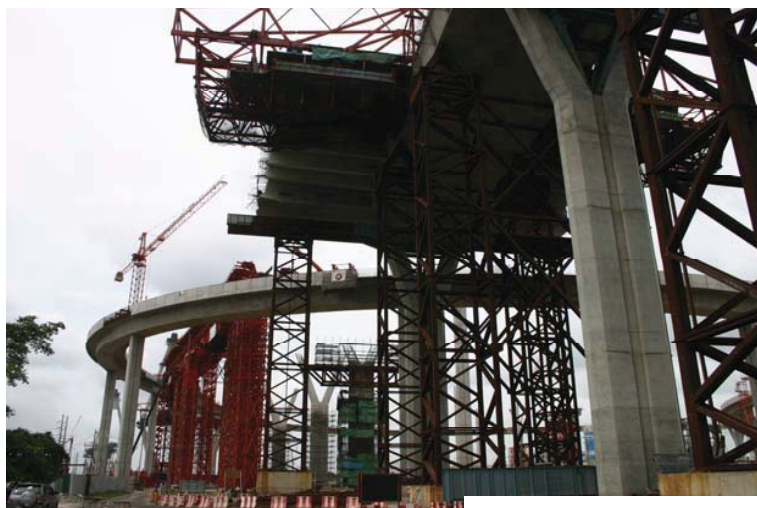
Construction of the Khlong Lat Pho intersection, Bangkok industrial ring road.
