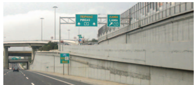
Figure 3: Sound barriers are a common measure to mitigate impacts of highways on the urban environment
