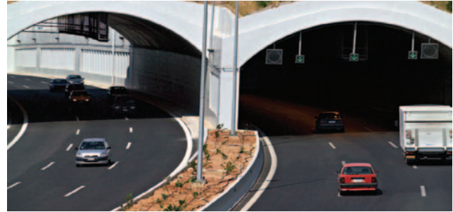
Figure 2: Cut and Cover helps to maintain a cohesive natural surface for flora and fauna.
