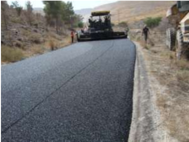
Pictures 1, 2: SMA overlaying job near Beit Shean with AMBS, wax modified PG 76-22 and Basalt aggregates (August 2010)
