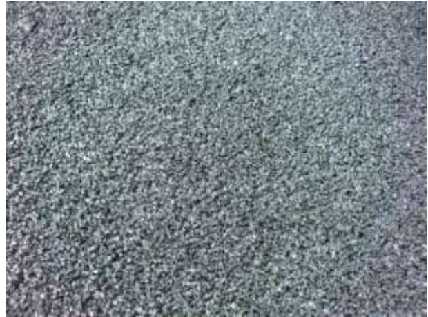
Pictures 1, 2: SMA overlaying job near Beit Shean with AMBS, wax modified PG 76-22 and Basalt aggregates (August 2010)
