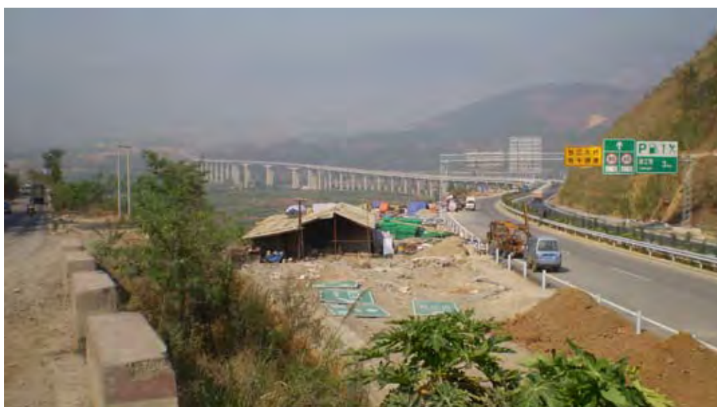
Baolong Highway construction almost complete, Yunnan Province, PRC
