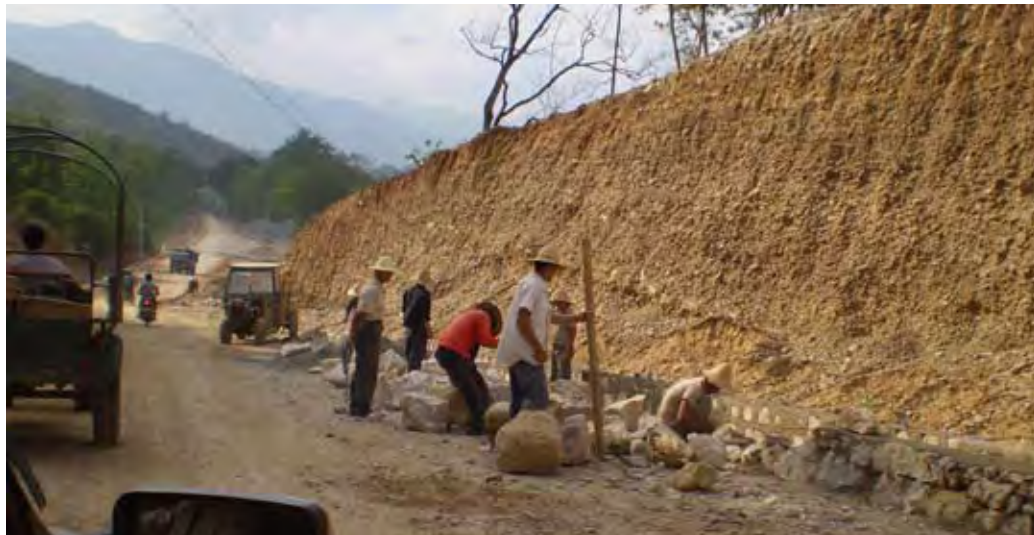
Work continues on access roads, Western Yunnan
