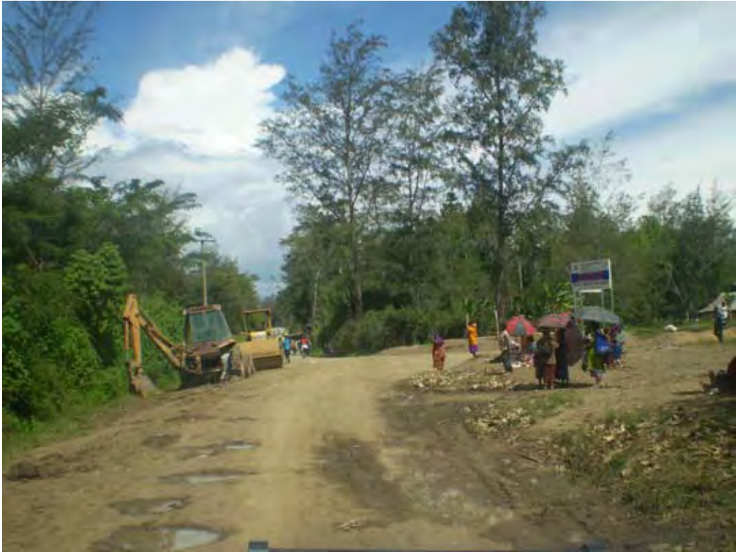
Road works, Western Highlands, PNG
