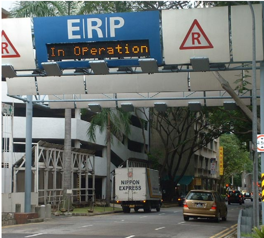
Figure 9 ERP Gantry Singapore. Karl Fjellstrom 2002, GTZ Urban Transport Photo CD
