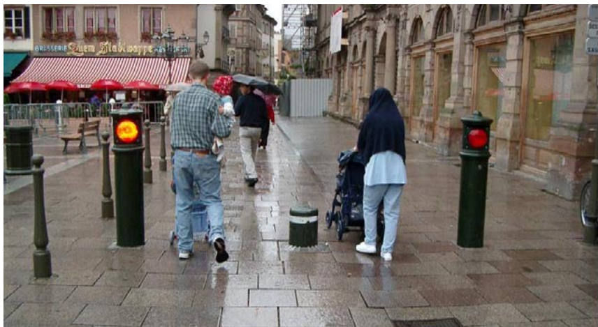
Figure 5 Concealable barrier for cars at the entrance to a car free zone, Strasbourg.
