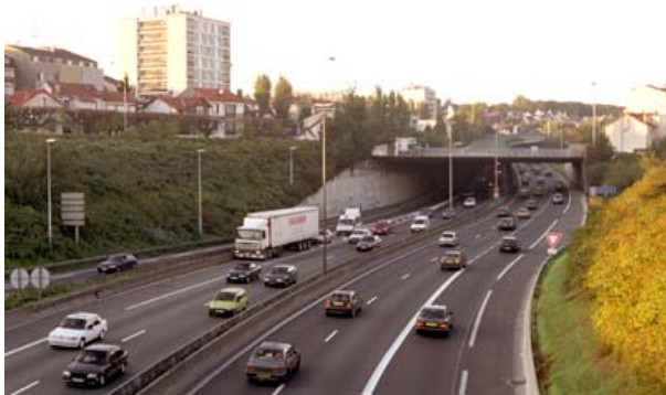
Picture 5: Traffic infrastructure in urban areas is very costly
