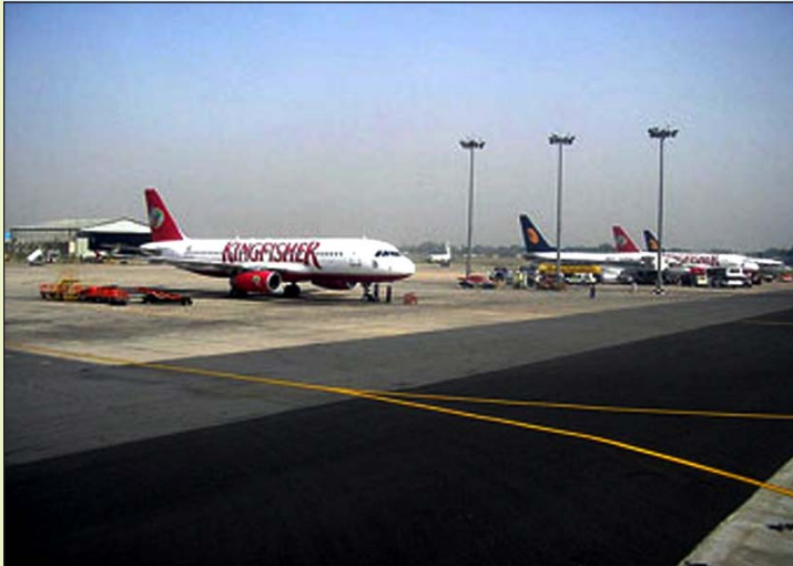
Design & construction management of airfield pavement upgradation at Bangalore
