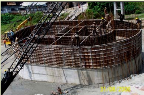
Consultancy Services for Jubilee Bridge (Substructure under construction)
