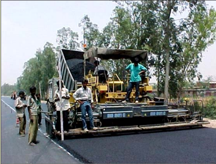
Construction supervision of four laning of NH-46, Tamil Nadu
