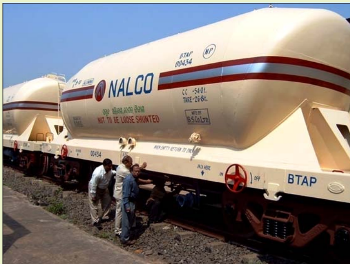
Operation & Maintenance of rail system at NALCO's S&P complex at Angul.
