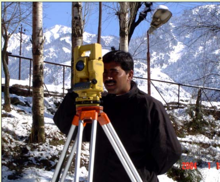
Pre-construction survey of new railway line from Katra to Srinagar – Baramulla via Qazigund in J&K
