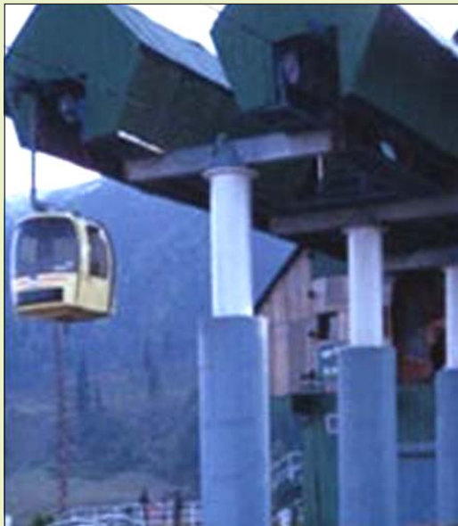
Project Management, Quality Assurance & Commissioning of Gulmarg Gondola ropeway.
