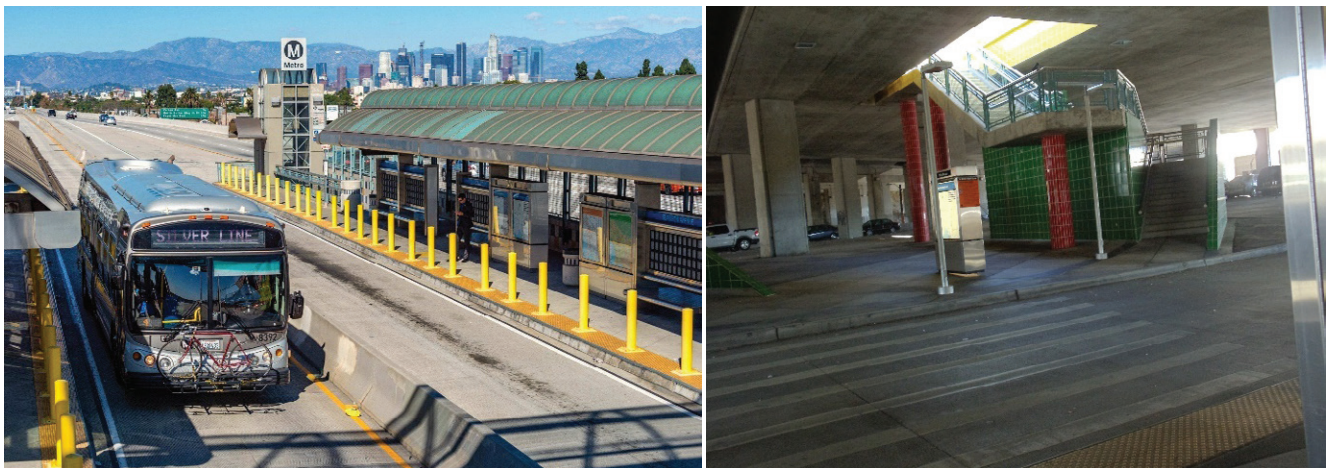
Access from below freeway: J-Line, LA Metro, showing elevated freeway median station (left) accessed from the local roadway below the freeway (right).
