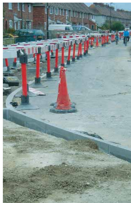
Construction at Abingdon, Oxfordshire
