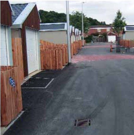
Telford completed cul-de-sac
