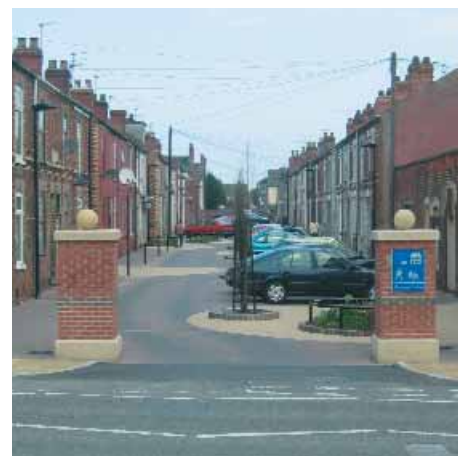
Gateway at Scunthorpe
