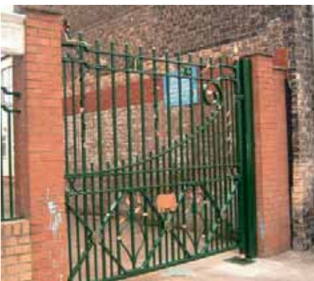
Hull gates – after
