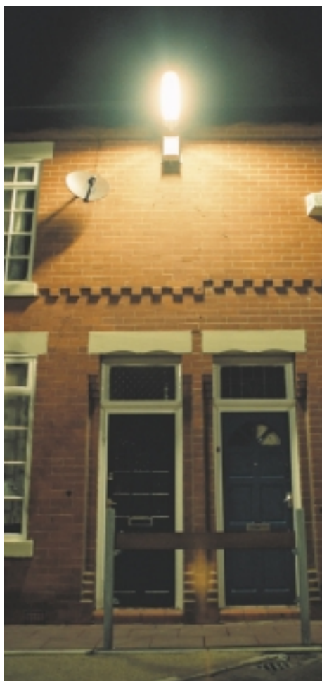
Lighting units mounted on buildings.
