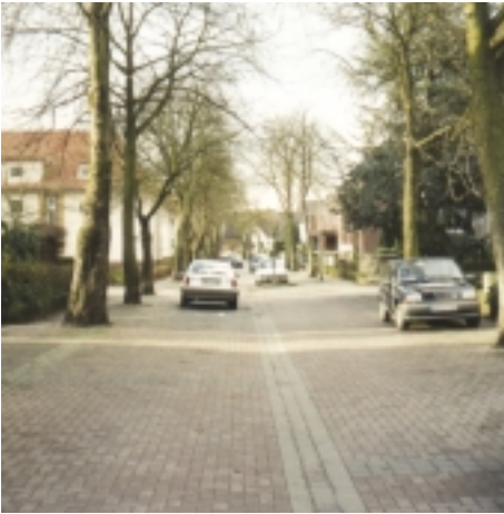
Shared surface with central drainage channel.
