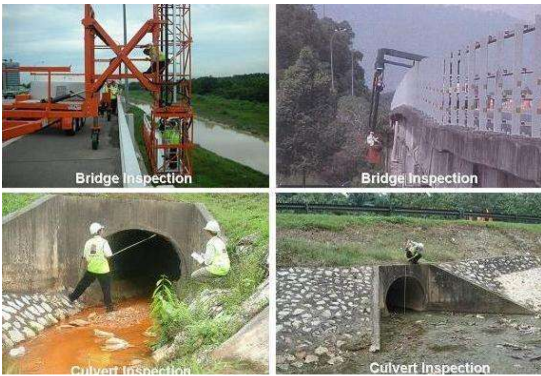
Plate 3 : Asset Condition Assessment of Bridges & Culverts
