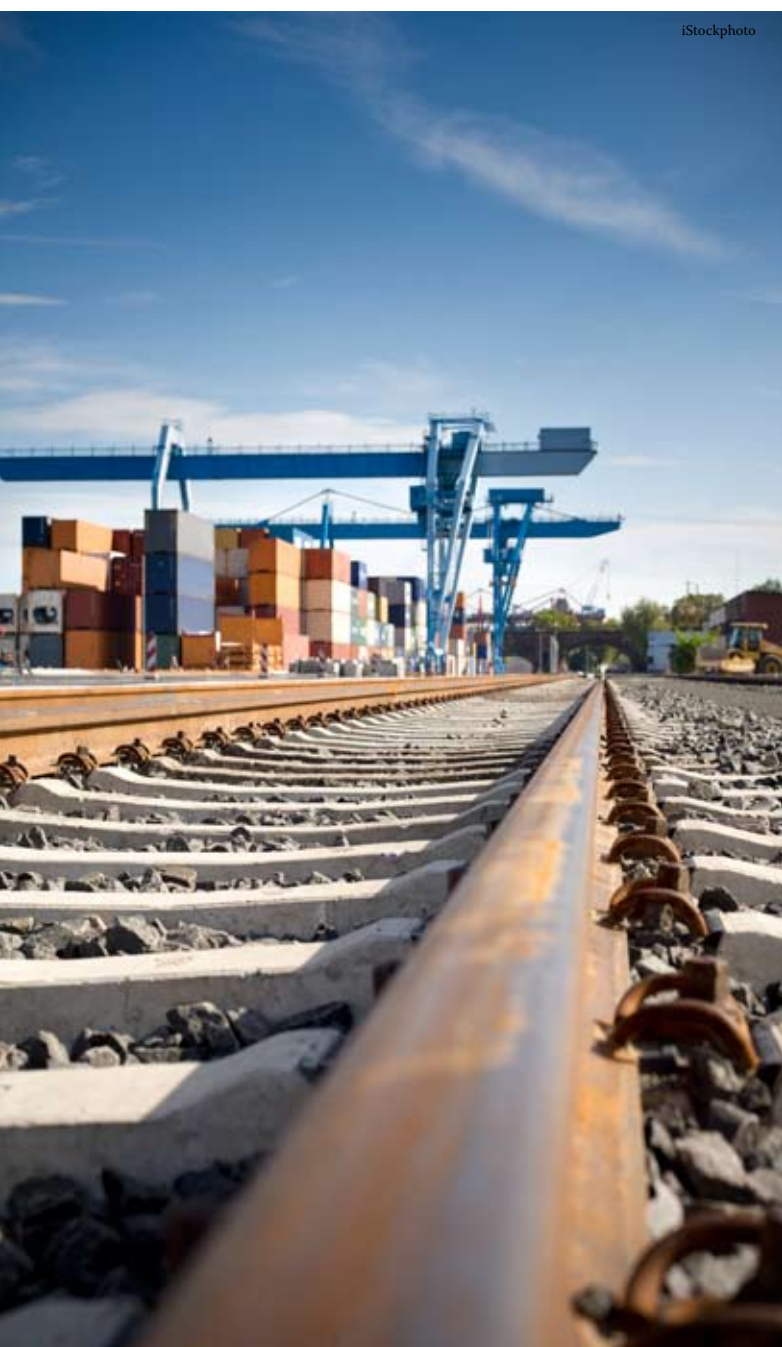
Container terminal Mainz, Germany features rail connections.
