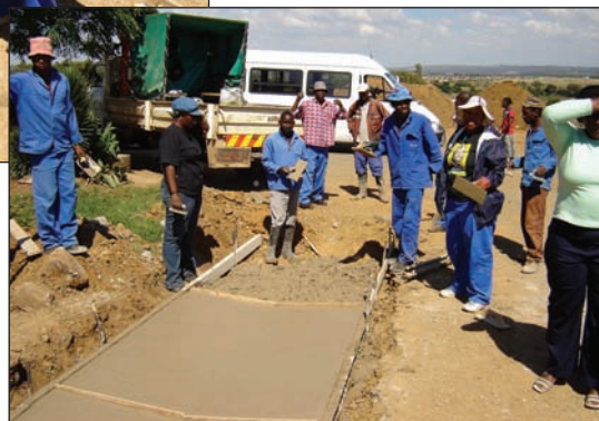
Another photograph of a labour-based construction project
