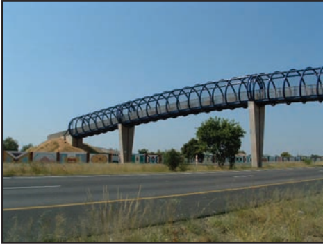
Innovative pedestrian bridge over freeway
