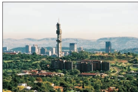
Tshwane Central Business Area
