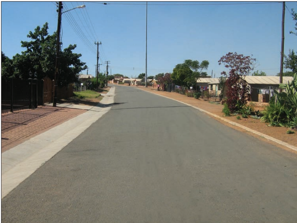
Residential township in Tshwane in a previously disadvantaged area, where the roads and storm water system has been upgraded.
