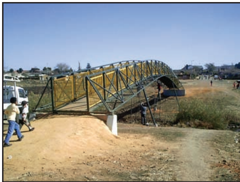
Lower-cost pedestrian bridge
