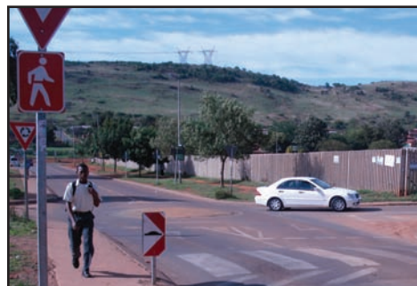
Mini-circle with raised pedestrian crossings
