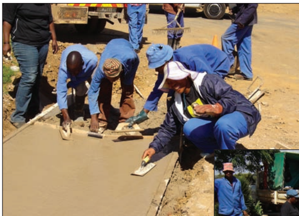
Labour-based construction involving community members
