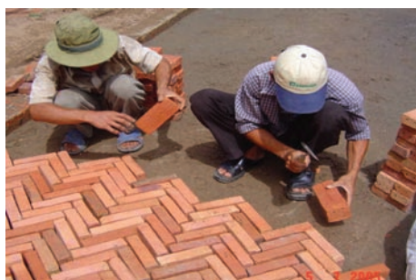
Laying bricks in 'herringbone' pattern between previously laid kerb edge restraints (bricks bedded and jointed in sand-cement mortar, on a conventional road base).
