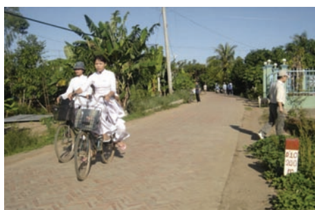
Completed brick paving road in service.
