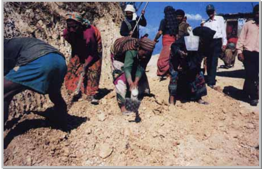
Photo 2503/10 – Palpa, March 1997 Labour intensive earth work excavation, Aarebhanjyang – Rampur road
