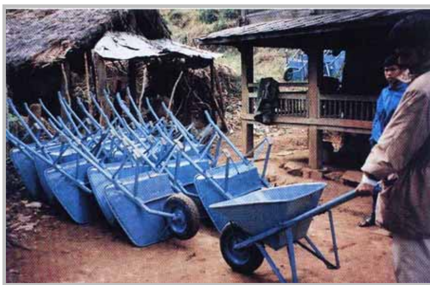
Photo 0622/24 – Gorkha, Dec. 1997 Store management of wheelbarrows at the construction sites
