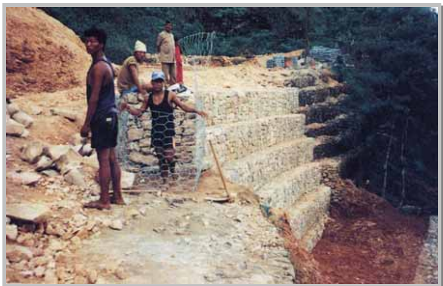
Photo 2474/37 – Syangja, 1997 Construction of gabion wall on the Naudanda – Karkinetta road
