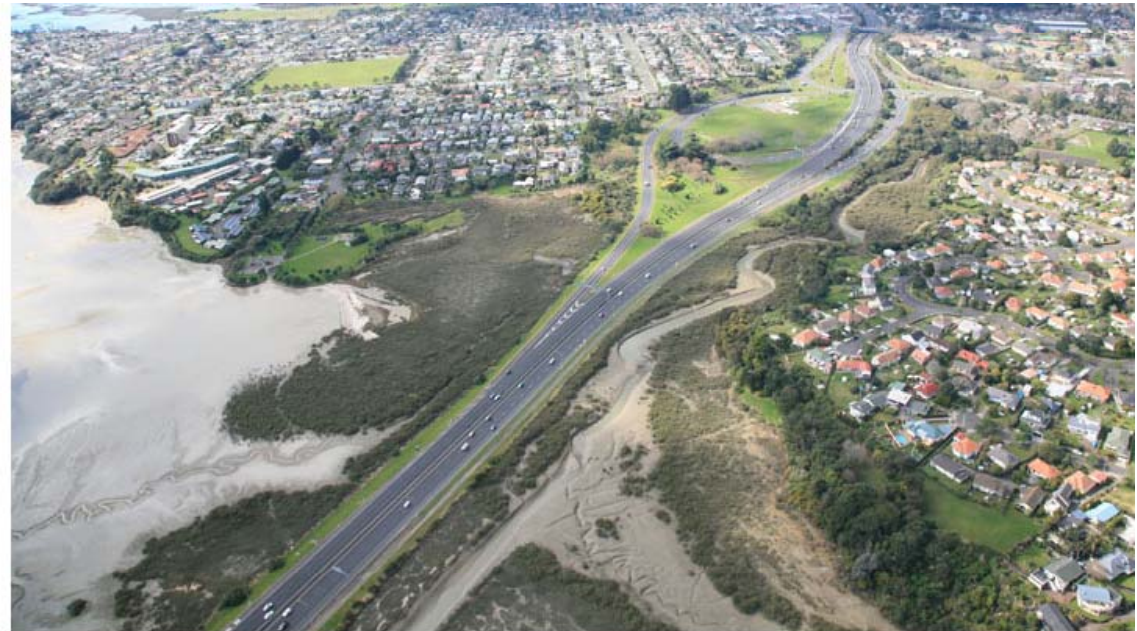
The Waterview Connection Application includes the work to extend SH20 and the capacity improvements to SH16 to Te Atatu.
